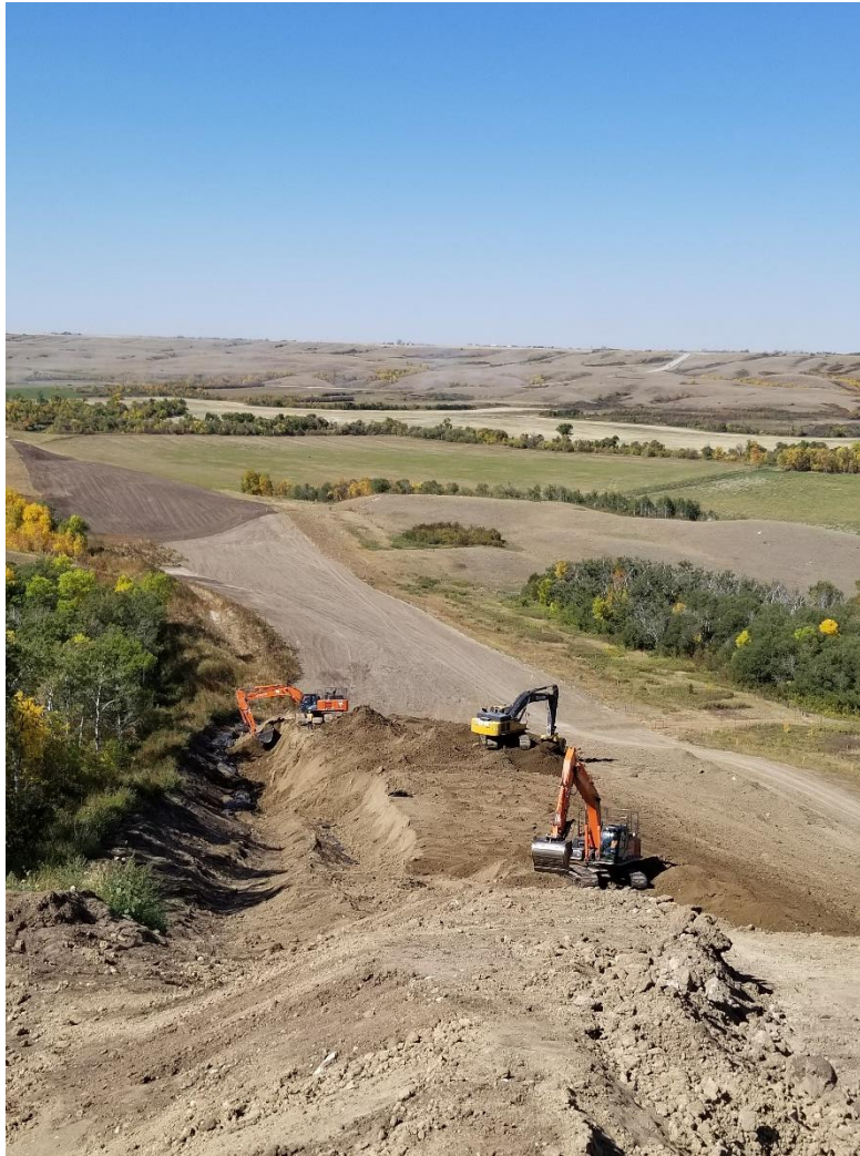
Qu'Appelle Valley Slope being put back, crew moving subsoil.
